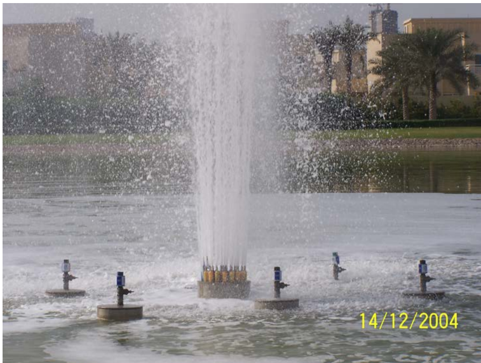
Installation of magnetic devices onto a fountain, Dubai
